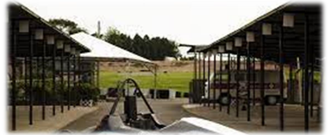
ECPA box installations
